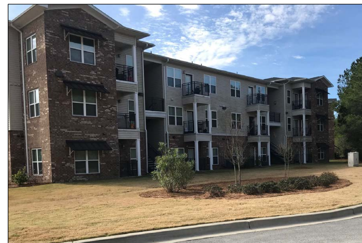
THE WATERS AT ST JAMES APARTMENTS
