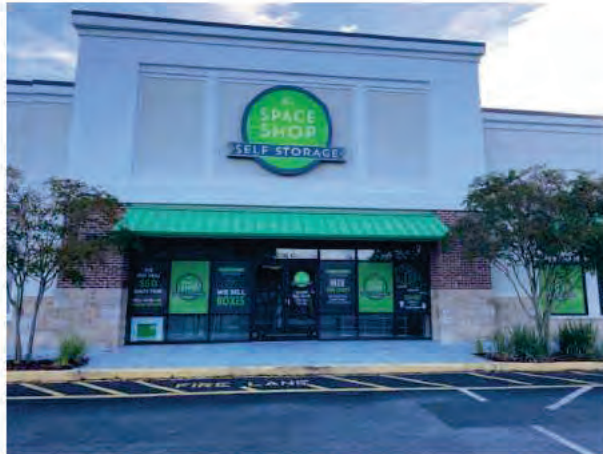
*EXISTING STORAGE SHOP VINYL TO BE REMOVED; SURFACE TO BE CLEANED FREE OF ADHESIVE
