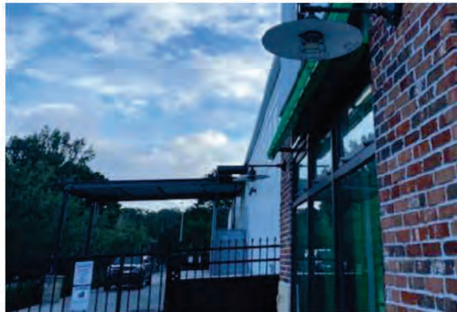
*REMOVE AND DISPOSE OF EXISTING SIGNAGE
