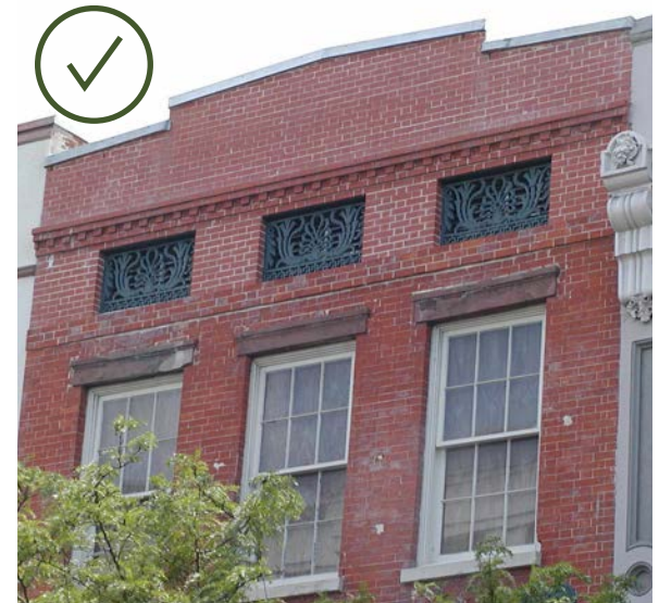
Because this buildings flat roof is screened by a parapet wall, it may be of any material.
