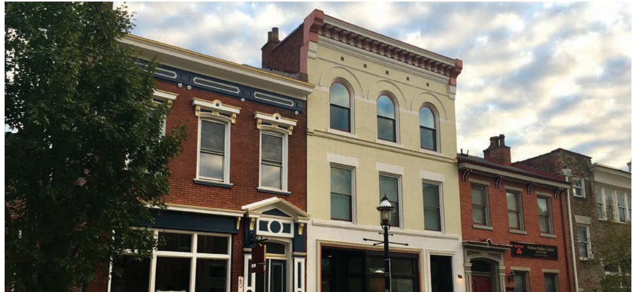
Example of buildings at varied heights.
