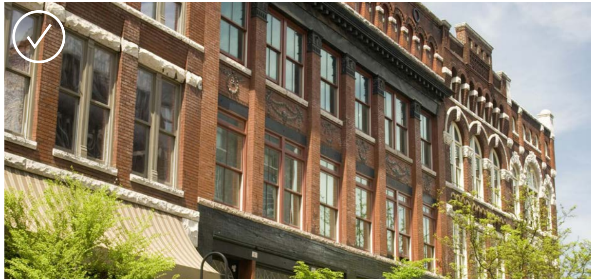
Unpainted brick, unpainted stone, and unpainted terra cotta are appropriate for the Central Creek District.
