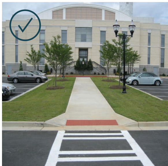
A walkway connects from the public sidewalk to the primary building entrance.
