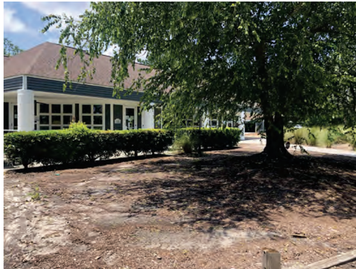
EXISTING REAR (EAST) FACADE
