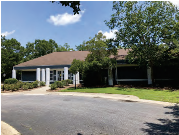
EXISTING FRONT (WEST) FACADE
