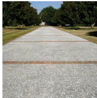
TABBY CONCRETE USED THROUGHOUT PATIO AND PAVED AREAS
