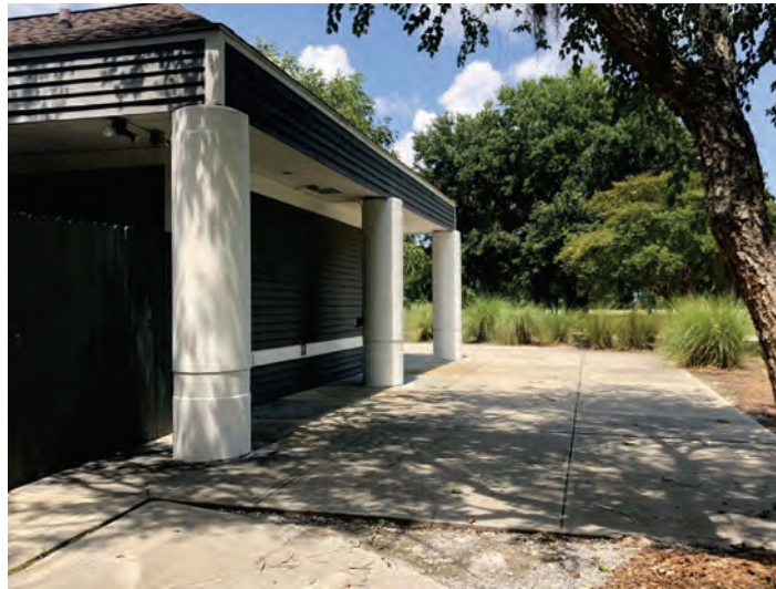
EXISTING SIDE (SOUTH) FACADE
