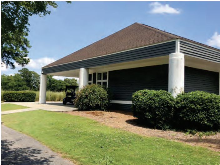
EXISTING SIDE (NORTH) FACADE
