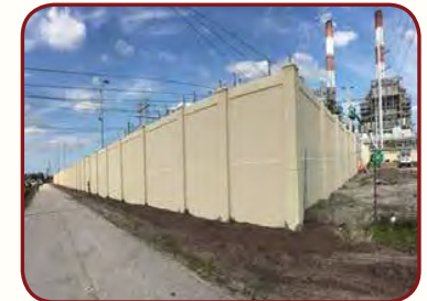
FPL Sub Station
