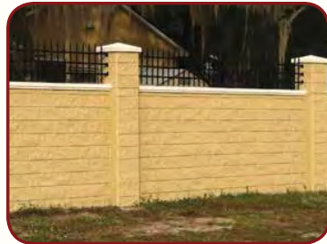
VA Hospital Perimeter Wall
