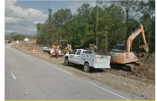
Construction of shared-use path on Henry E. Brown, Jr. Boulevard between Liberty Hall Road and Red Bank Road.
