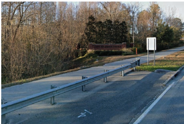
Shared-use path parallel to US-52/ Goose Creek Boulevard provides Goose Creek residents access to North Charleston's Wannamaker County Park.
