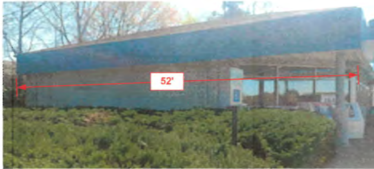
EXISTING BUILDING – LEFT SIDE
