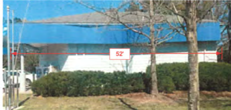
EXISTING BUILDING – RIGHT SIDE
