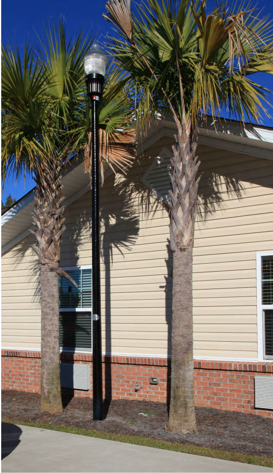
PHOTO OF PROPOSED SITE LIGHTING
