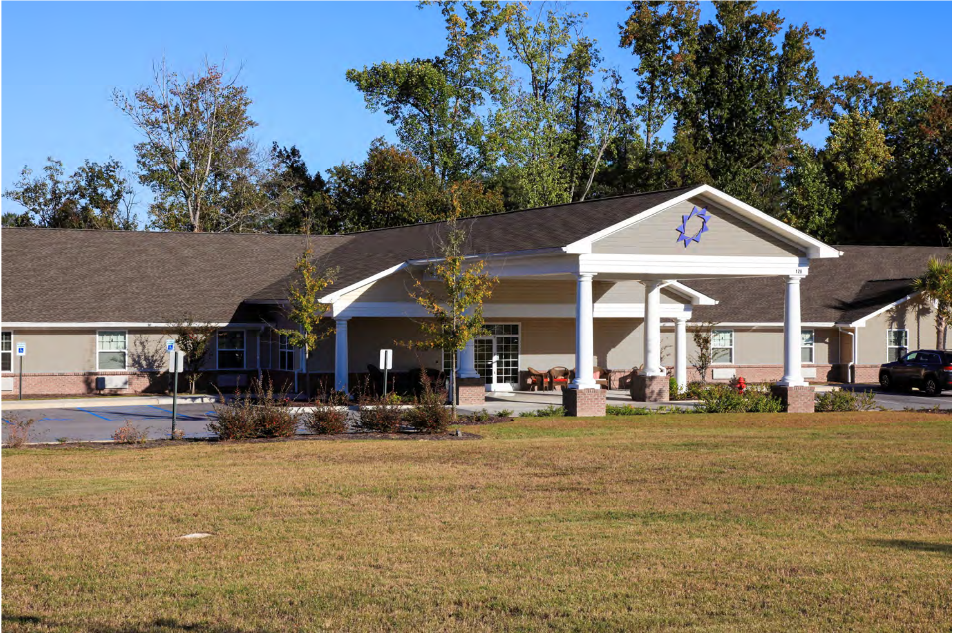
Color Photo of Similar Building with proposed color scheme Agape House of the LowCountry
