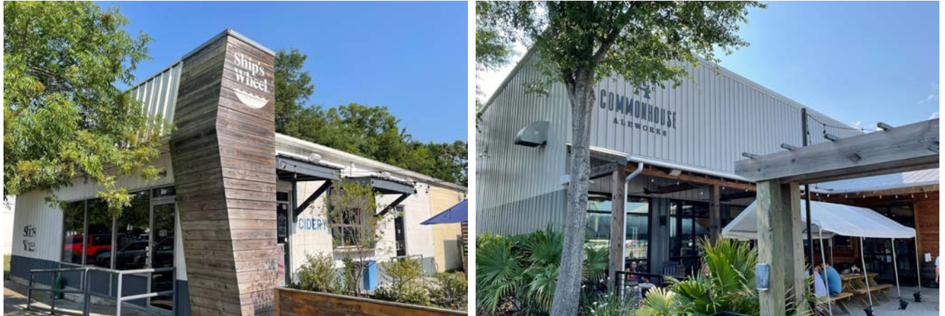
Example of corrugated metal, wood, awnings and two-tone paint schemes to create simple, attractive facades
