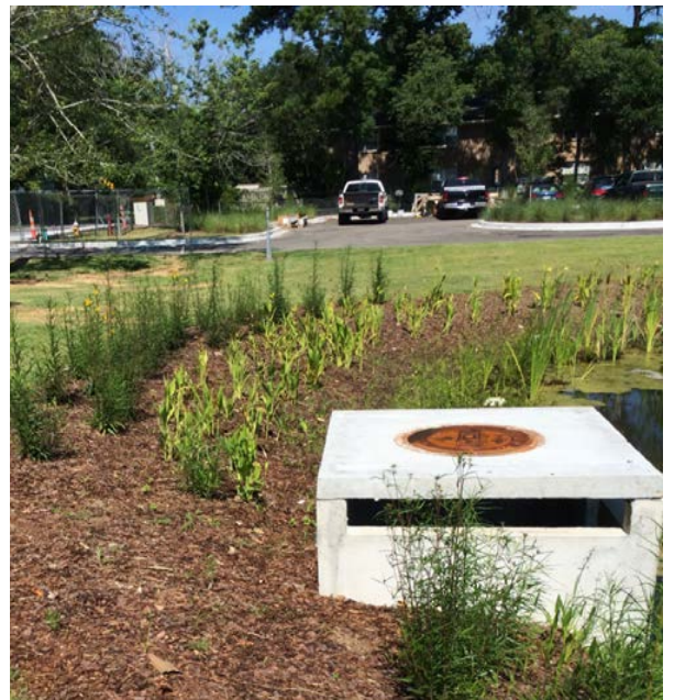
Example of retention ponds and edges
