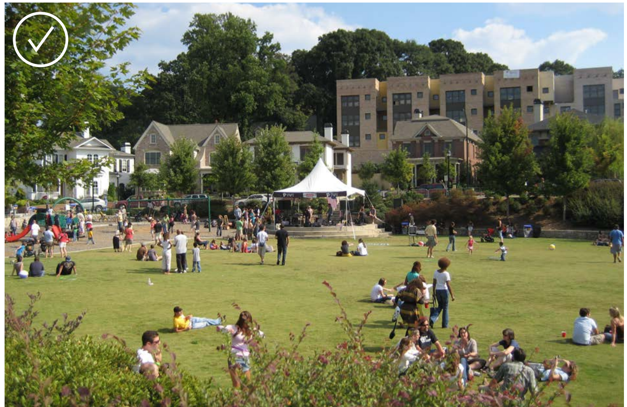
This park doubles as the development's stormwater detention facility.
