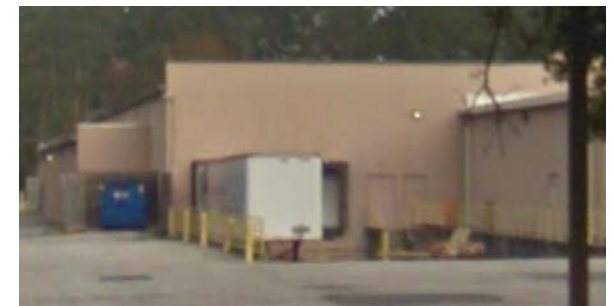
○ VIEW OF REAR
