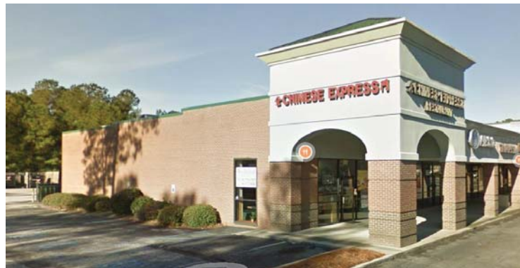
○ SOUTH EXISTING FAÇADE
