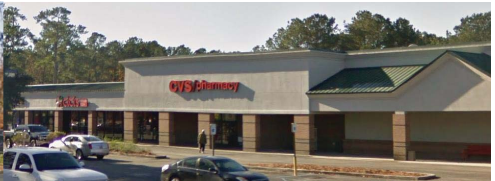
○ CENTER-LEFT EAST FAÇADE
