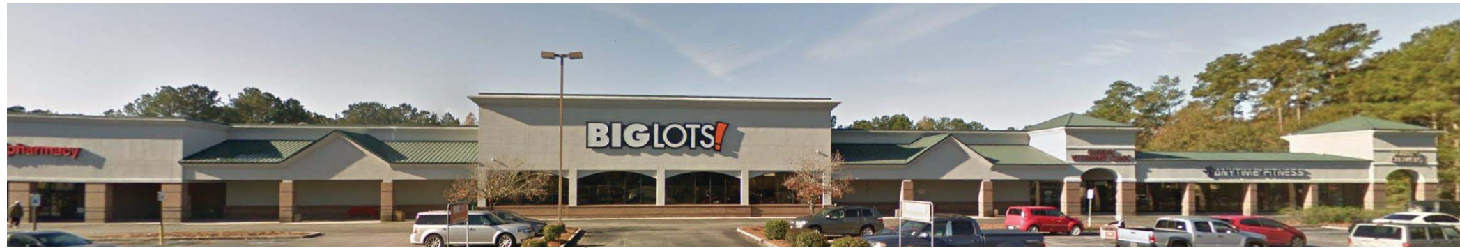
○ CENTER & RIGHT EAST FAÇADE
