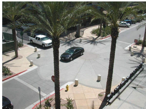
Raised intersection in Phoenix, AZ
