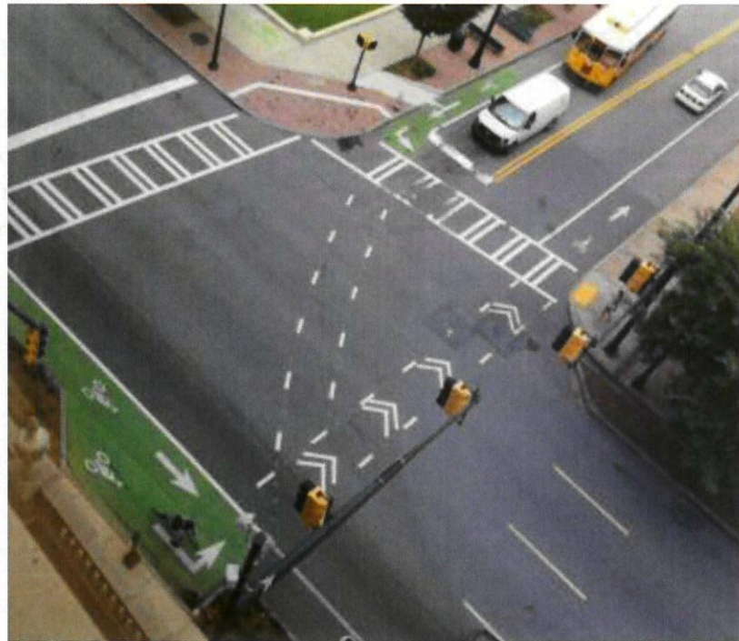
Examples of different pavement markings and signals for bicyclists at intersections (Photo: W. Peachtree St., Atlanta)
