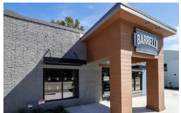
Example of high-quality composite wood used as accent material for entry cover.
