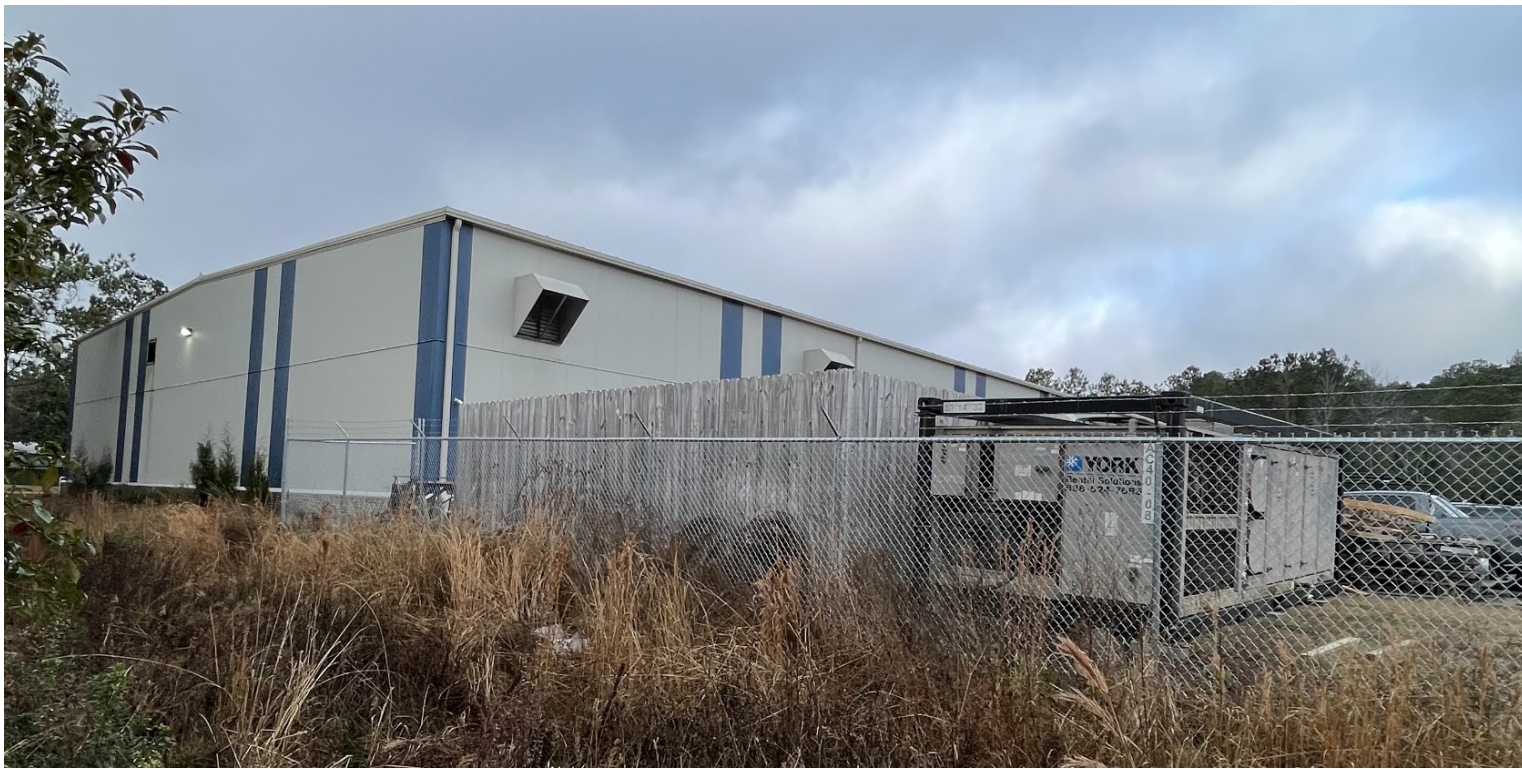
View North of existing C.R. Hipp building
