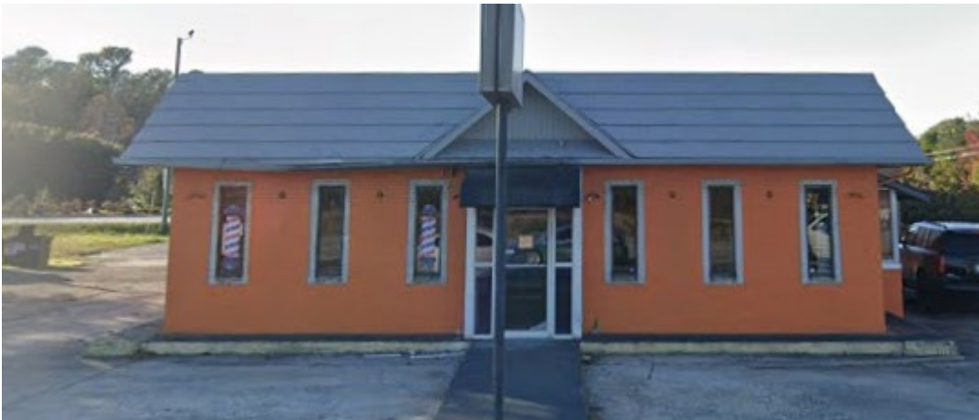
Figure 2: View of structure from parking lot on N. Goose Creek Boulevard side.
