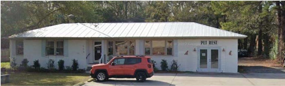
Figure 1: Primary structure on lot.
