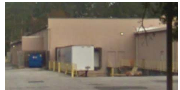
○ VIEW OF REAR
