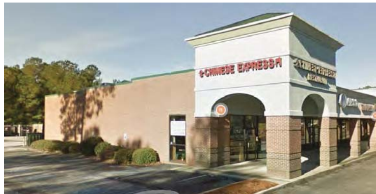
○ SOUTH EXISTING FAÇADE
