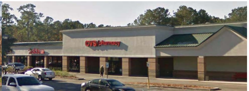
○ CENTER-LEFT EAST FAÇADE
