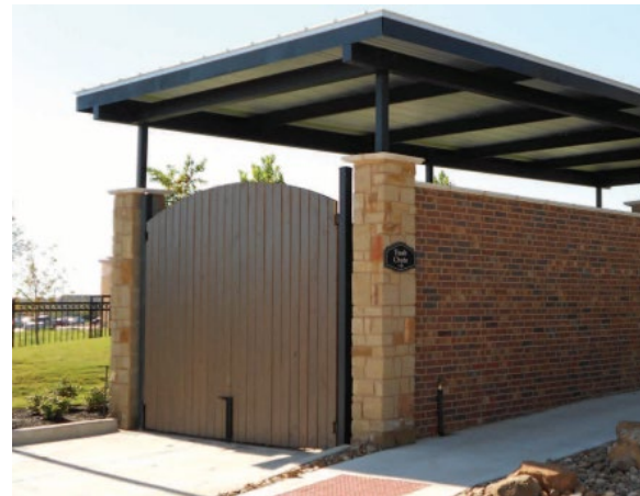
Example of refuse collection screening.
