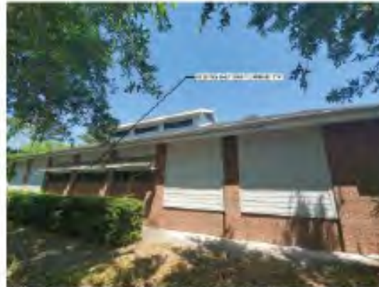
EXISTING BUILDING FACADE FACING BEN SAWYER
