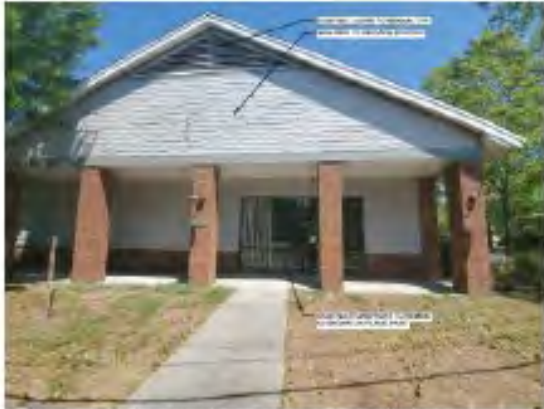
EXISTING BUILDING FACADE FACING BEN SAWYER
