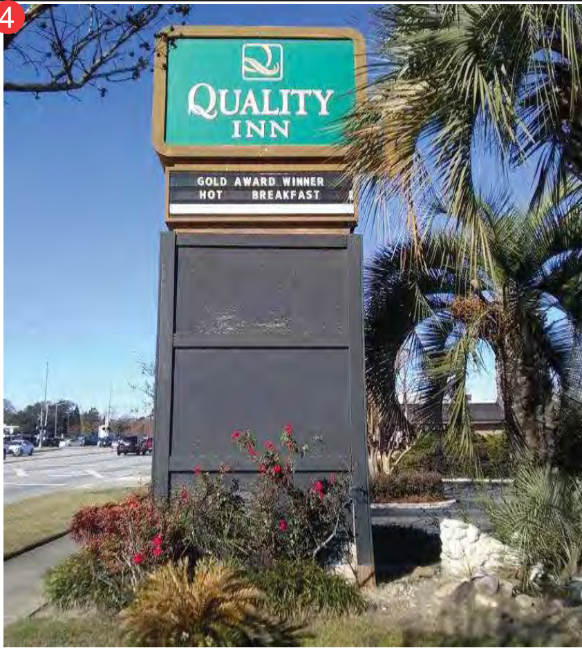
EXISTING 5'0 1/2" X 7'6" PYLON SIGN AT 19'4" OAH
